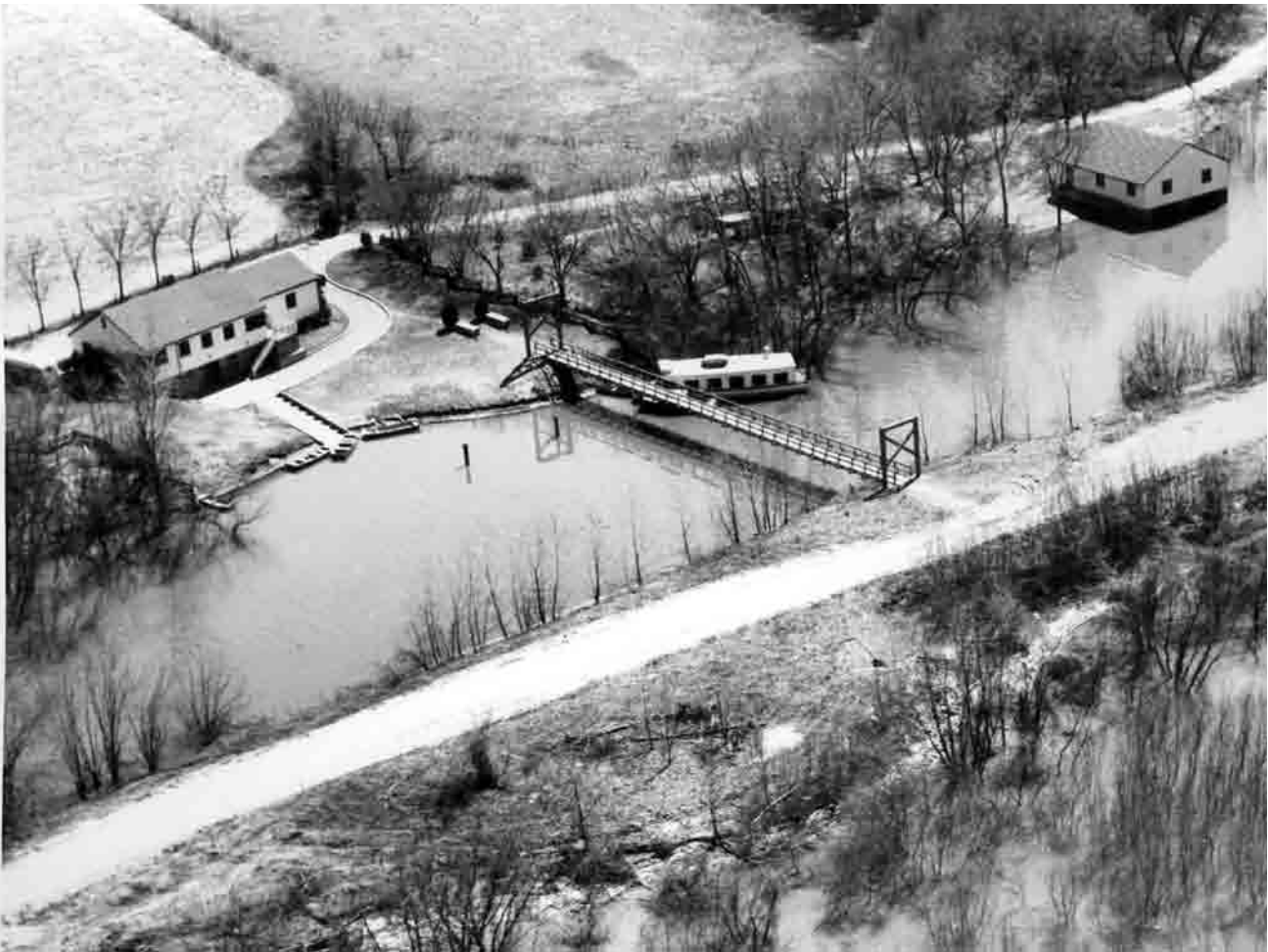
During the depression years of the 1930s, the federal government established work programs that made possible a variety of construction projects. The Survey made use of that opportunity to construct a building to house the Havana Station. The frame structure was completed in 1940, a mile or so from the site on Quiver Lake where Forbes had established the station in 1894.
